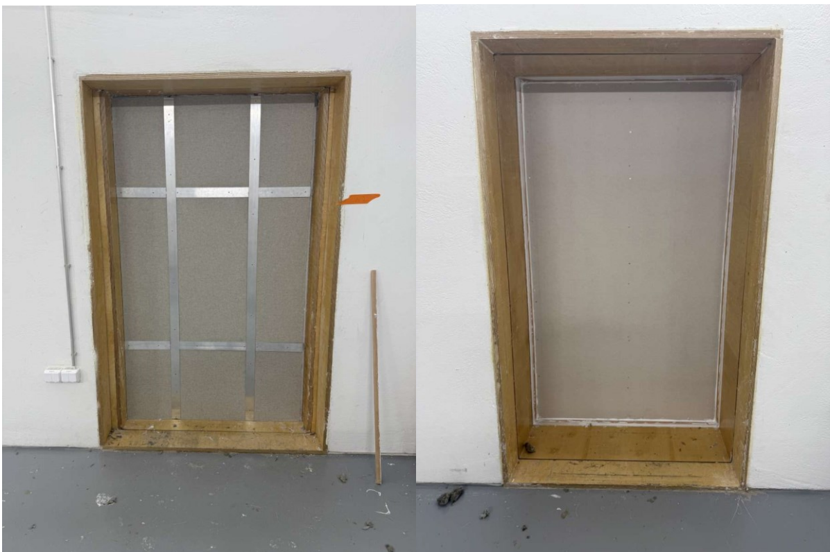
Figure A3.3. The Wall 2 installation into the test opening. The image on the left is viewed from the source room. The image on the right is viewed from the receiving room.)
