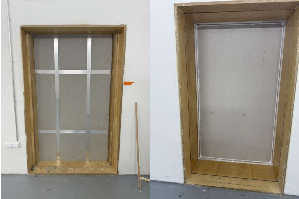
Figure A3.2. The Wall 1 installation into the test opening. The image on the left is viewed from the source room. The image on the right is viewed from the receiving room.
